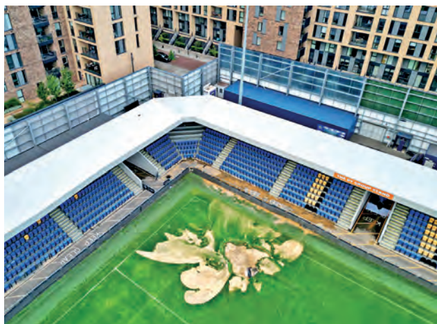
London, UK A drone view of a sink hole caused by heavy rainfall, on the pitch at the Cherry Red Records Stadium, home of AFC Wimbledon football club in south-west London.
