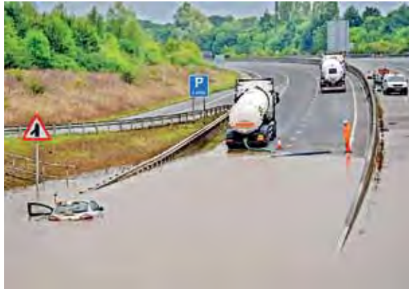
Marston Moretaine, England A car remains submerged in flood water on the A421 in Bedfordshire as tankers continue to pump out the water. Wet weather will persist across parts of the UK.
